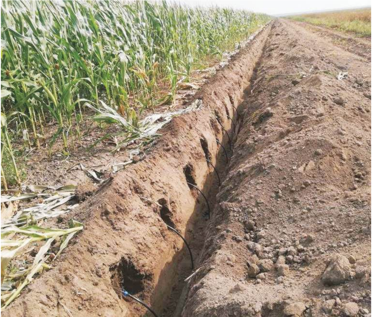
Buried drip irrigation
